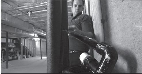
Paul Laferriere , HVAC Technician, Custom Mechanical Services
